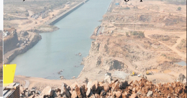
Navi Mumbai International Airport Project Site after blasting operations
